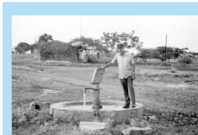
Water flowing from broken handpump
