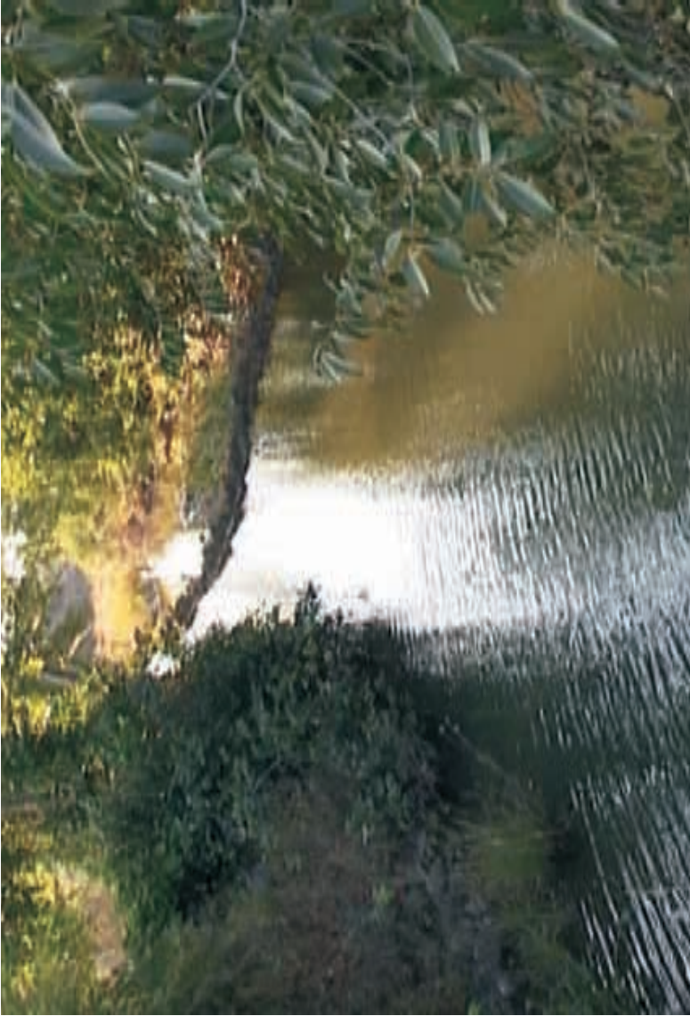
A konda – water storage and diversion weir
