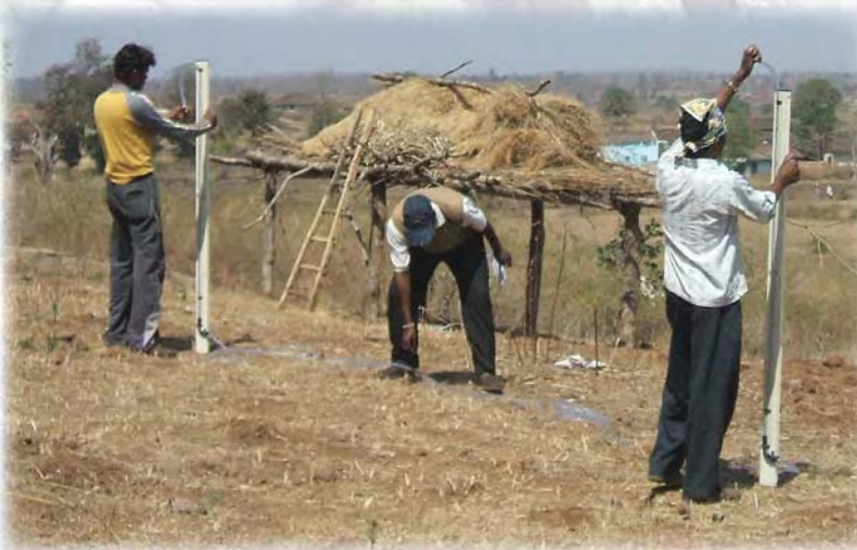
Slope Identification and Layout Marking
